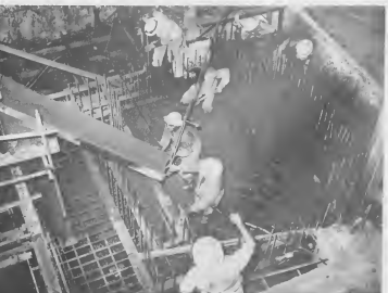
WORKMEN SPREAD approximately forty yards of concrete into the area that will eventually become the foundation for a new turbine in No. 2 Powerhouse. The first pour of concrete formed the mat. There is other pours before the foundation in the Powerhouse pump room is ready for the 7500 KW turbine.
